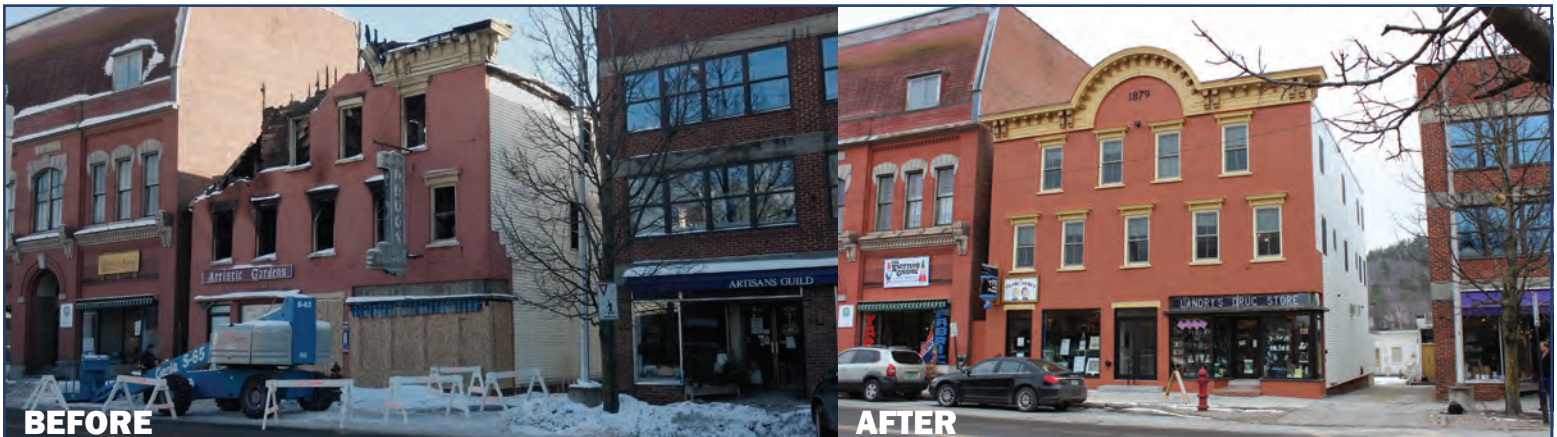
After a fire just before Christmas 2012, the Landry Block (1879) on Railroad Street in St. Johnsbury was saved and rehabilitated with the aid of tax credits in 2013. Not only was the historic character of the building preserved, code improvements mean the two commercial units and four apartments are now fully accessible.
